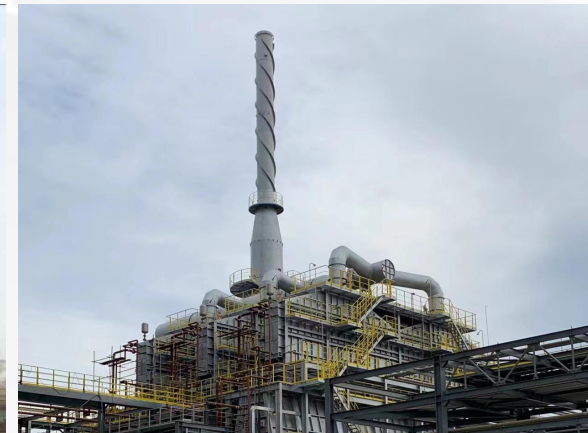
针状焦加热炉 Needle coke heating furnace
