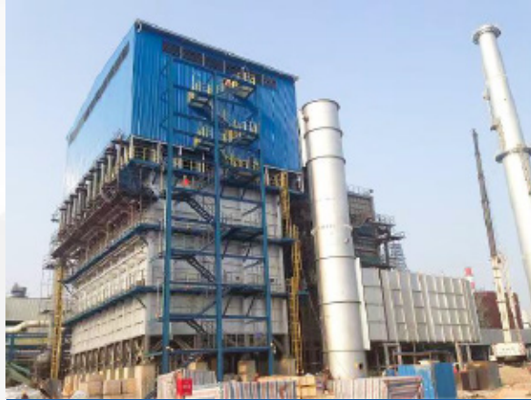
Hydrogen producing reformer
